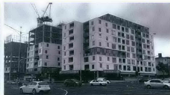
3. MULTISTOREY APARTMENT DEVELOPMENT AT 410 BURWOOD HIGHWAY
