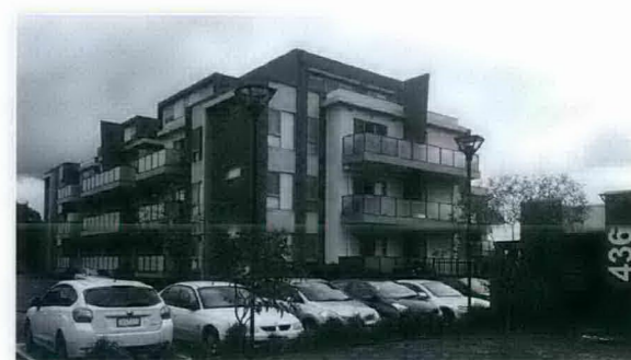
1. MULTI STOREY APARTMENT DEVELOPMENT AT 436 STUD ROAD
