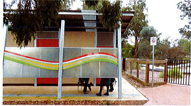
Tim Neville Arboretum: Use of screening allows for high casual surveillance with chosen colour palette giving site a strong sense of place and design with doors facing a common walkway
