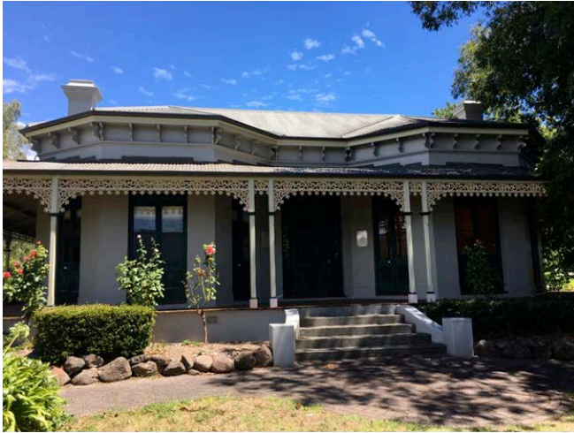
View of the front of the homestead. Note French doors and roof profile, steps and rocks to garden bed
