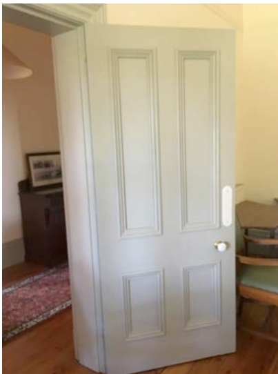
A typical four panel door
