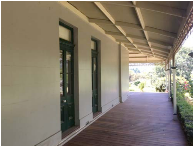
View of verandah (Note: recent verandah floor)
