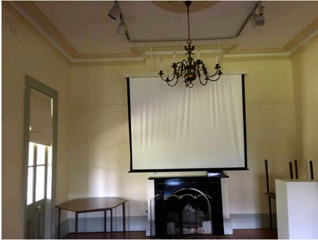
View of room on left of hall showing original fireplace and typical cornice, skirting and architrave detail
