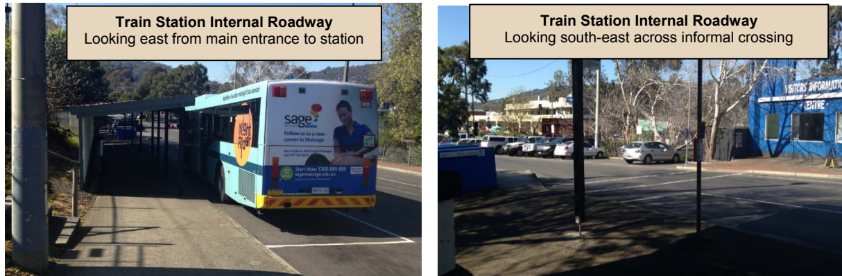
Figure 28: Bus Stops at Upper Ferntree Gully Train Station
