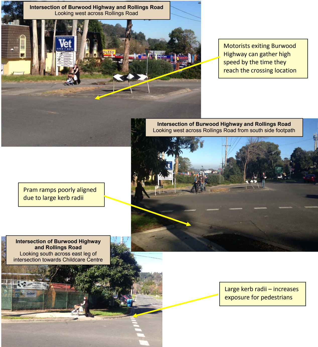
Figure 25: Intersection of Burwood Highway and Rollings Road – Existing Conditions
