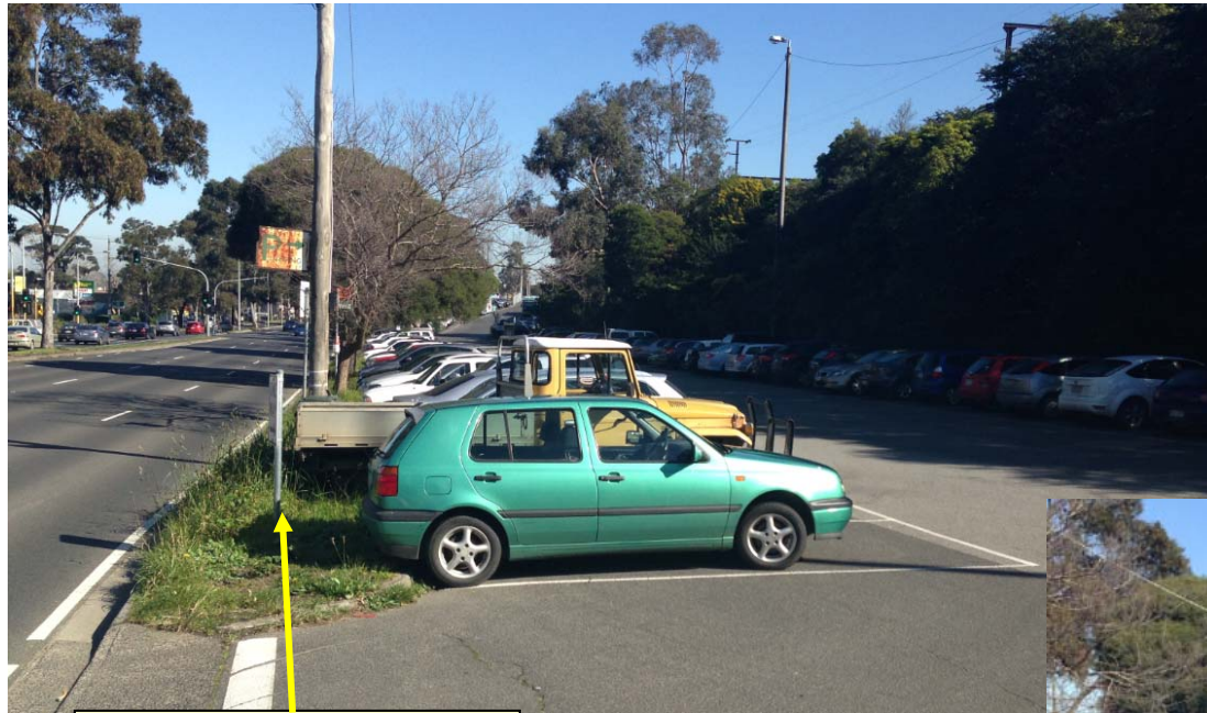
Figure 42: East end of Train Station Car Park – Construction of Footpath
