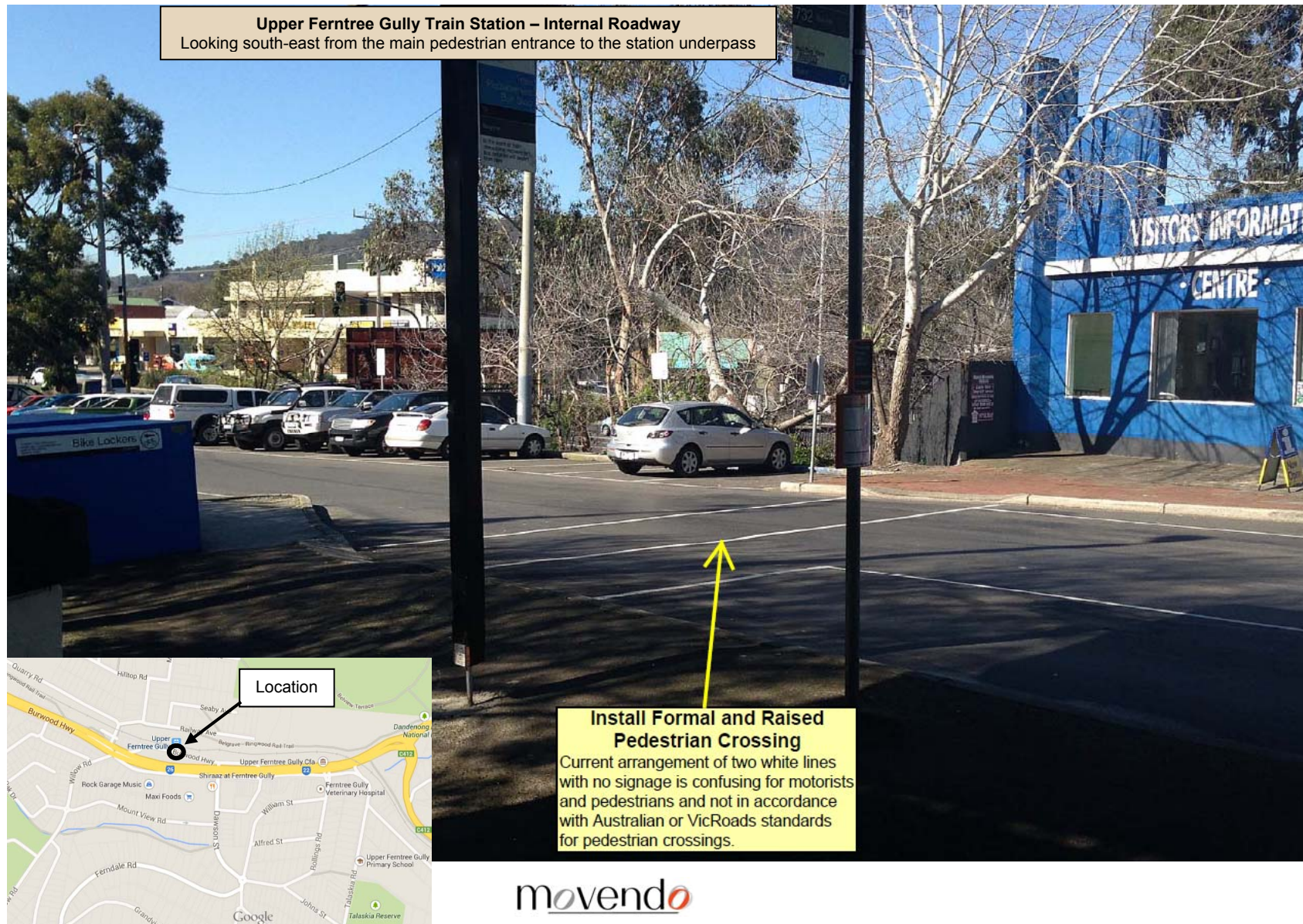
Figure 46: Train Station Car Park – Install Raised Pedestrian Crossing outside main entrance to connect Bus Stops
