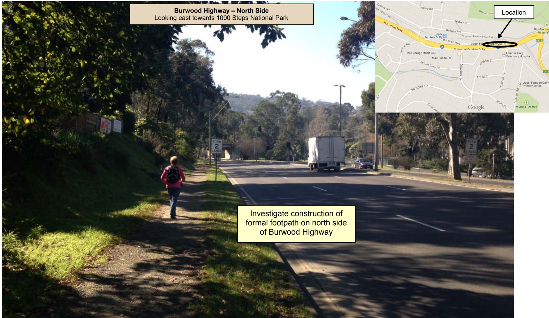
Figure 43: Burwood Highway – North Side: Between Station Car Park and 1000 Steps National Park - Construction of footpath
