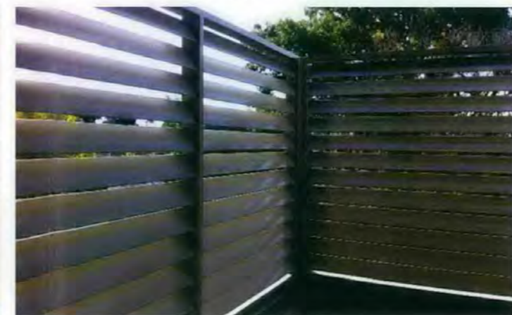
MATERIAL- POWDERCOATED METAL LOUVERS
