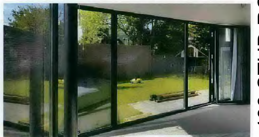
MATERIAL- POWDERCOATED ALUMINUM WINDOWS
