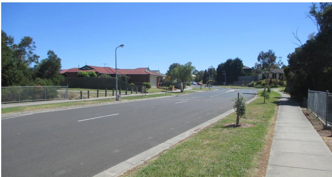
Figure 3 Typical road asset under Council's responsibility
