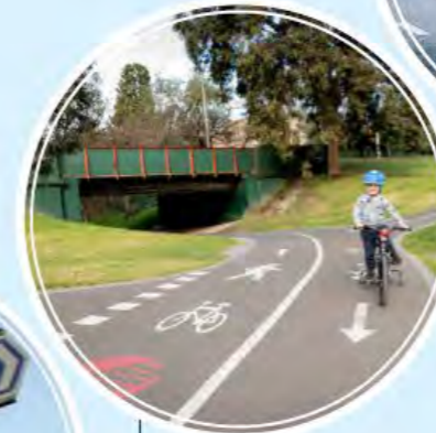
1.5 Improved underpass safety for cyclists and pedestrians.
