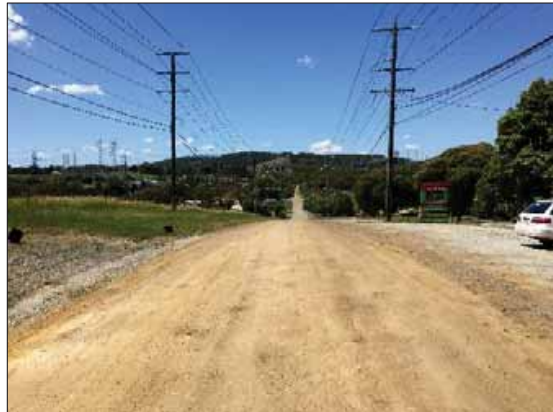
Figure C4: Police Road (view east)
