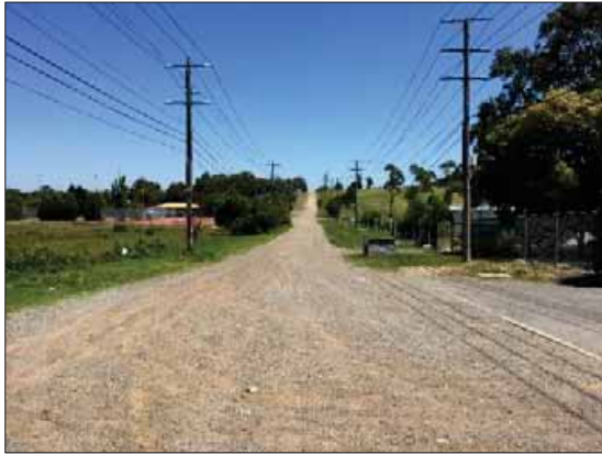
Figure C1: Police Road (view west)
