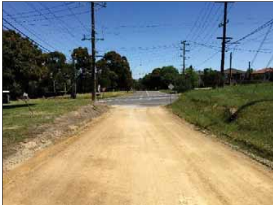
Figure C3: Police Road (view west)
