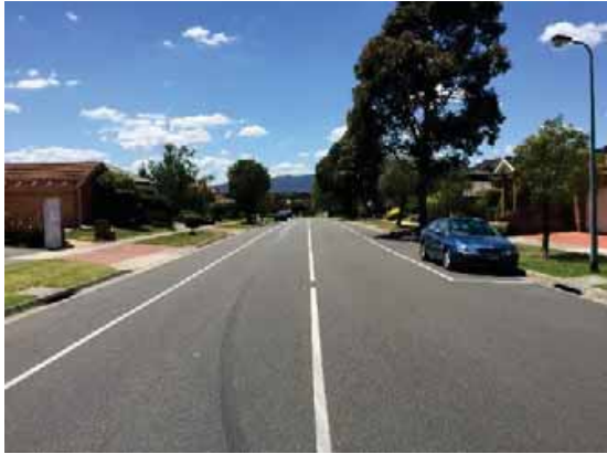
Figure C7: Liberty Avenue (view north-east)
