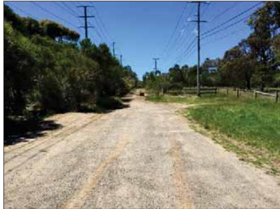
Figure C2: Police Road (view east)
