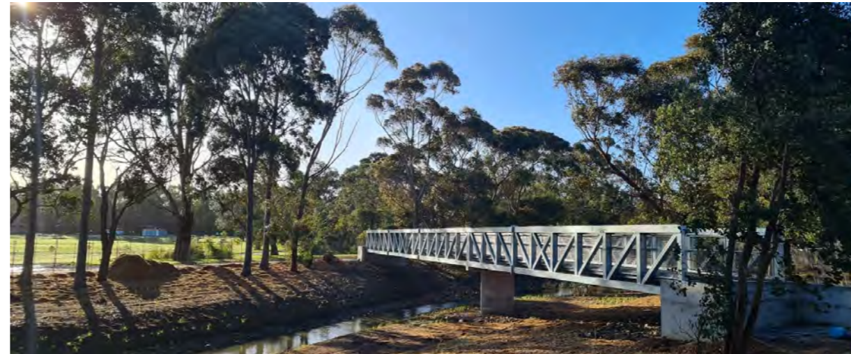
Figure 10: View of the new pedestrian bridge on Blind Creek, 2024
