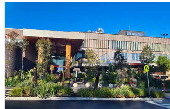
Figure 8: North facing façade of Westfield Knox, 2024
