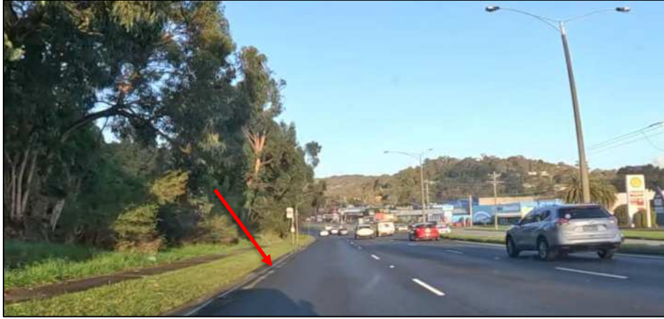
Burwood Highway eastbound - looking east (red arrow indicates approx. location of start of deceleration lane)
